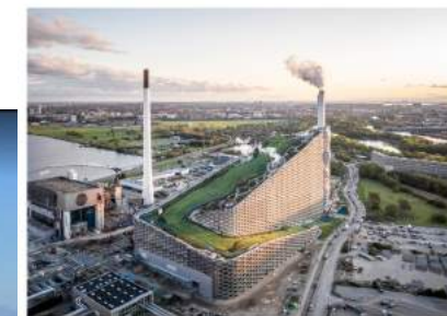
The 1,450-foot artificial ski slope is covered in synthetic grasses that aim to provide the same friction as a lushly greened slope (though might be a little rougher on the skin). Business Insider
